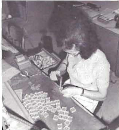
Kathleen Lucier is shown assembling coils into cups. The coil is placed over the centerpost of cup, covered with a washer. The leads are attached to the pins, and bent over the washer and the lead wires soldered to the terminal pins.
